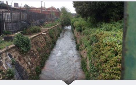
Canalised Jukskei River (Gauteng)
