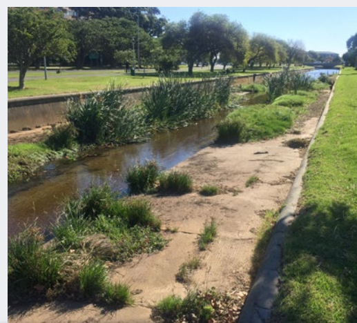
Establishment of indigenous riverine vegetation along the Liesbeek Canal, Cape Town. The vegetation creates desirable aquatic and marginal habitat – but its implications for flooding are untested
