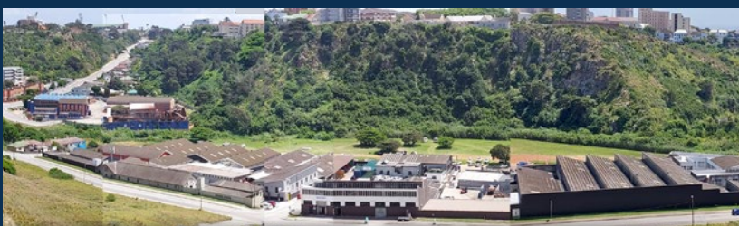
Construction of bridges, factories and buildings on the lower Baakens River floodplain
