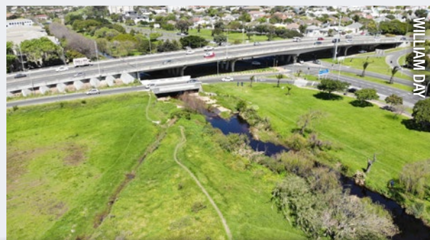
Flood flow diversion channel excavated into the Liesbeek River, Cape Town.
