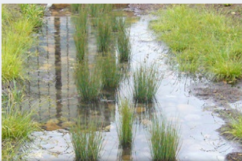
A rain garden installed to intercept runoff in an urban area.
