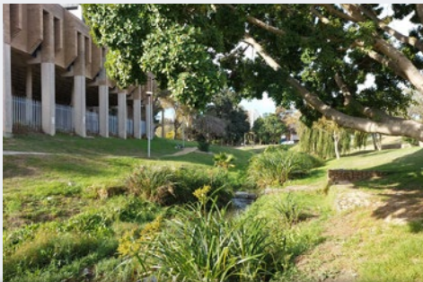
Buildings constructed on the Elsiekraal River floodplain.
