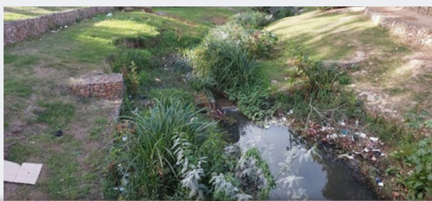
Flood banks can be set back from the channel to create space for high flows and flooding.
