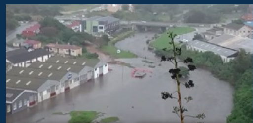
The damage caused to the Baakens River floodplain, and infrastructure, inundated after floods.
