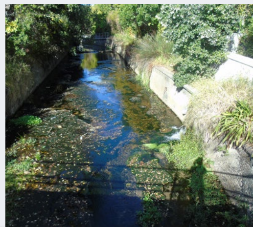
Planted riverine margins create cooling and riverine shading without impacting on river flood lines
